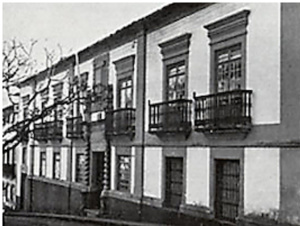
The House before having been renovated
