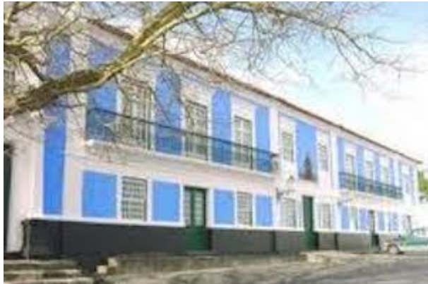
Solar da Madre de Deus (Manor of the Mother of God) - Today hosts the official residence of the Minister of the Portuguese Republic
